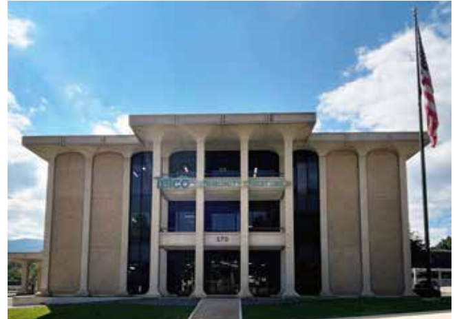
Waynesville Professional Building 370 N. Main Street
